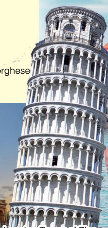
Leaning Tower of Pisa
